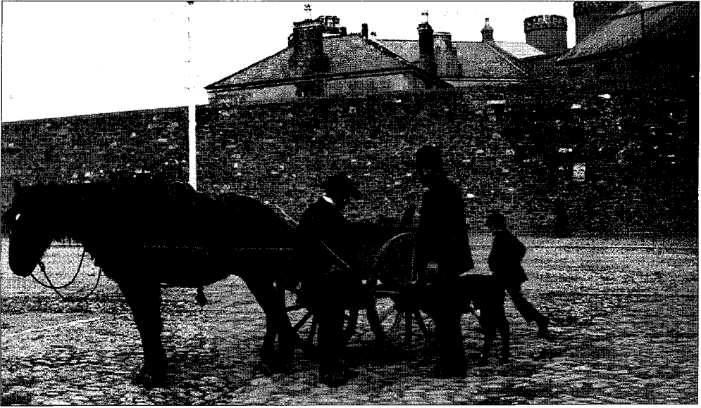
Picture of part of the last gaol erected in 1861-62, from the mouth of the Mayor's Walk. Note the condition of the street surface, the rough and uneven cobblestones – an everyday scene before the era of tarmacadam.
